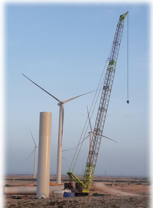
AEPL Project Turbine Erection in Progress
